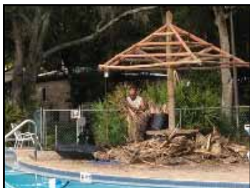
Thatching Removal
